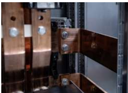
Detail kast-kastverbinding
