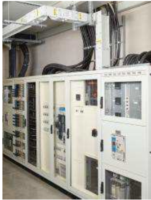
Connection of unibar H to unimes H
