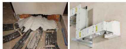
Cable laying (left) versus unibar H (right)
