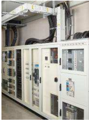
Connection of unibar H to unimes H
